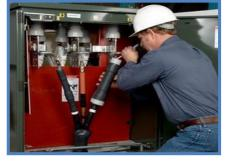
Cable terminations and joints form the weakest link in any distribution system. Also, a failed joint in an underground distribution system is much more difficult to locate and repair compared to any similar problem in overhead distribution systems. This means that we should do our utmost to achieve a good joint or termination, which can give years of trouble-free service.
